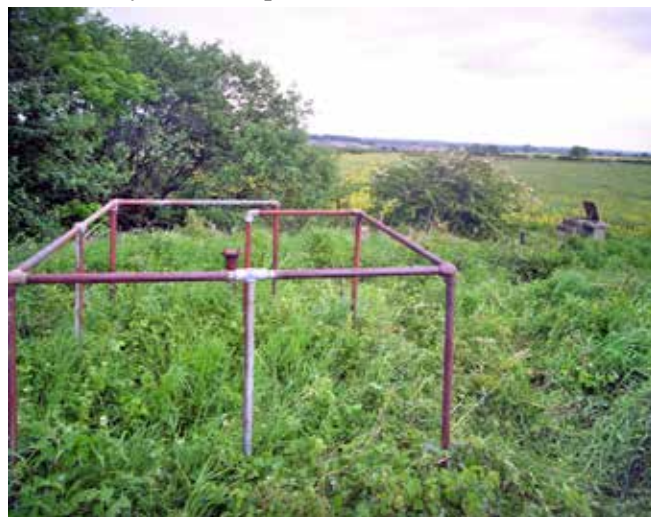
The conventional post is seen to the right. The railings are a simple aircraft observation post built on top of the Battle Headquarters. The FSM pipe is seen behind the railings, another is seen next to the underground access hatch. Photo Nick Catford
